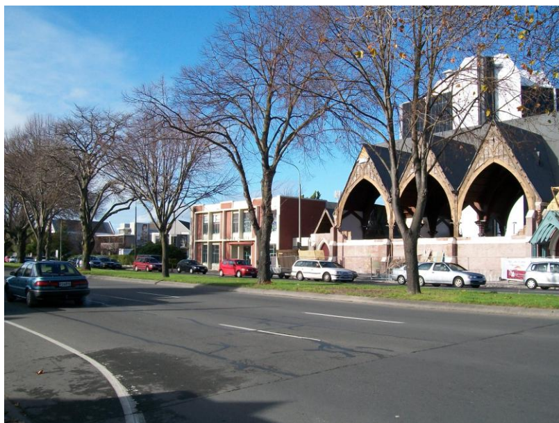
LifeLine Christchurch and LifeLine National office building survived whilst the Knox Church tumbled.
